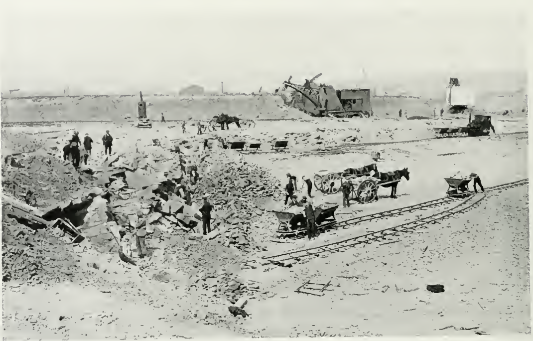
EXCAVATIONS AT LYNESS IN CONNECTION WITH THE BUILDING OF THE WHARF.
